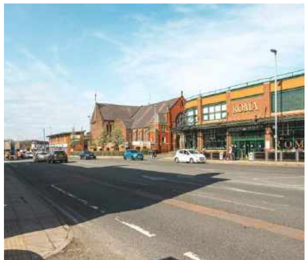
Width of carriageway creates unpleasant pedestrian environment
