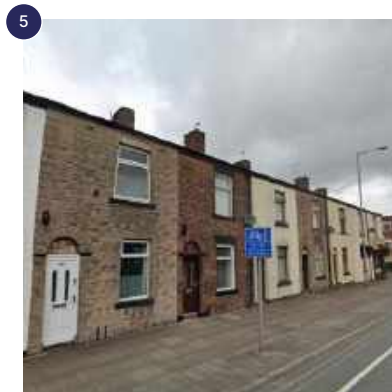
Ground floor frontage activated by residential entrances
