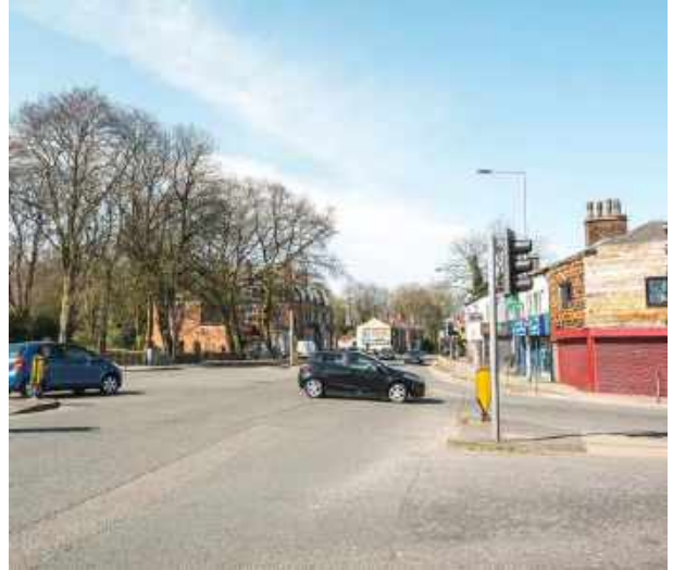
Carriageway dominates the environment
