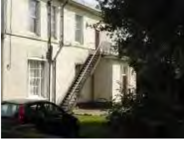
Intrusive Fire Escape at Summerseat House
