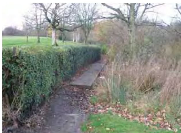
41: Path leading down from Bury New Road is in poor condition
