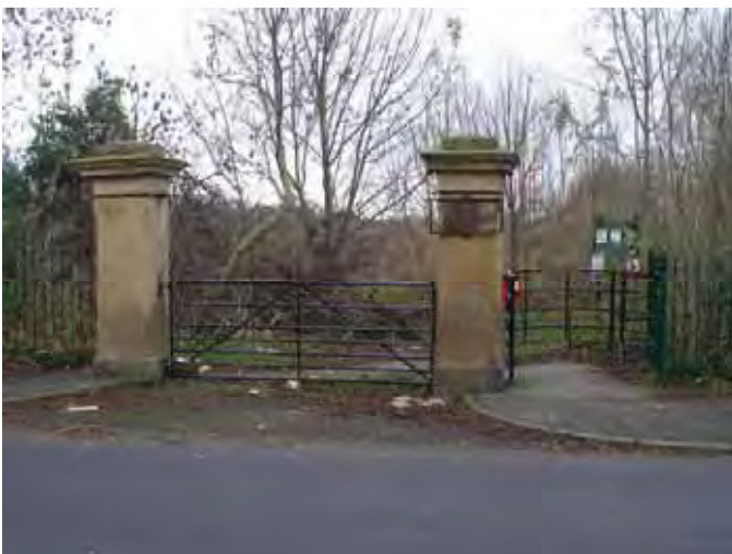
52: Entrance to Gardener's Mount in poor condition
