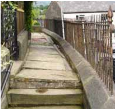
Fig. 36: Steps and railings on Tanners Street
