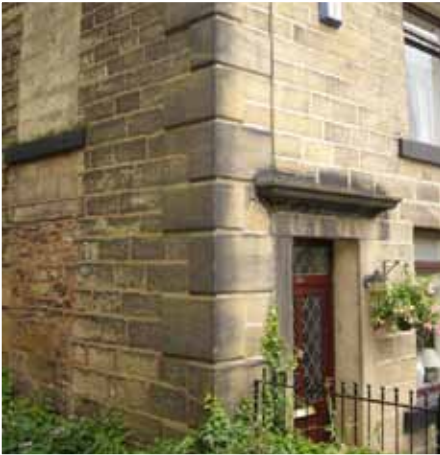
Fig.78: Chamfered quoins and door detail on a Tanners house
