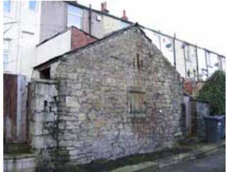
Fig. 18: An outhouse to rear of Victoria Street
