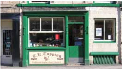
Fig. 33: Intact butchers' shop window at Number 11 Bolton Street, with sliding sash, halved door and transom ventilator
