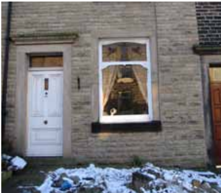
Fig. 25: Terraced house on Peel Brow with original sash windows and panelled door
