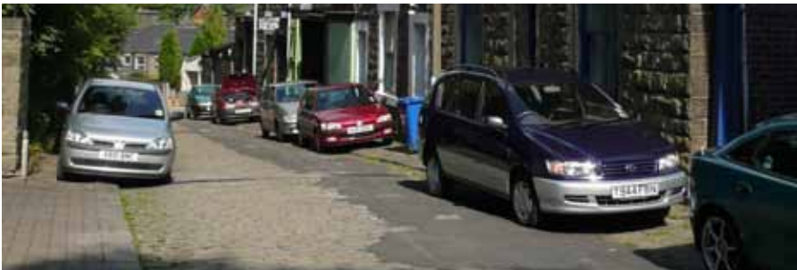
Fig. 57: Traditional setts contribute to the character of the street scene, but need careful repair - Paradise Street
