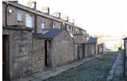
Fig. 35: Intact rear lane with setted surface and stone outhouses behind Crow Lane
