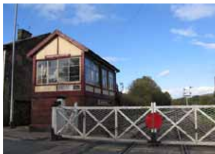
Fig. 22: 1938-9 signal box and level crossing
