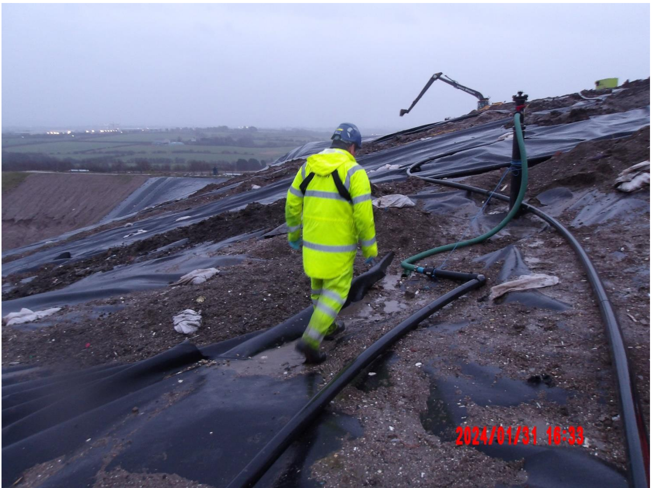
Picture above shows: An Environment Agency landfill officer inspecting the integrity of the capped area and gas management system following increased complaints the day before.
