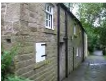
Cottages on Holcombe Old Road in Local Stone and with Coal Door
