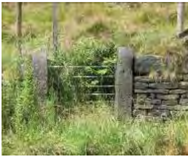
Traditional Stone Wall and Gateposts
