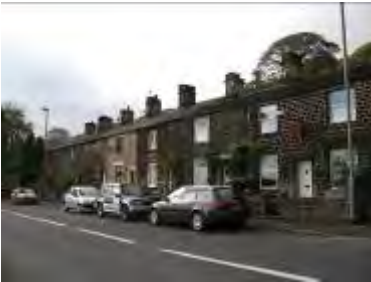
Ivy Cottages with Different Door Replacements and Wall Treatments
