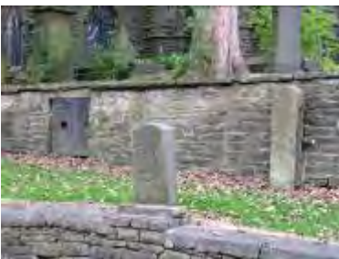
Coal Door in Church Wall
