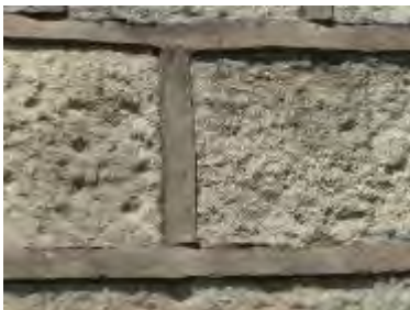
Use of Cement Mortar
