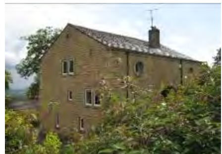
Rear of Plant Barn after Conversion
