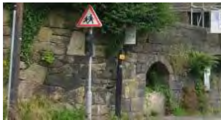
Water Trough and Retaining Wall on Helmshore Road
