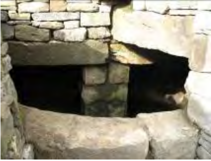
Stone Water Tank, Helmshore Road
