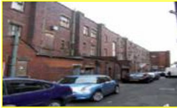
Poorly designed service corridor
