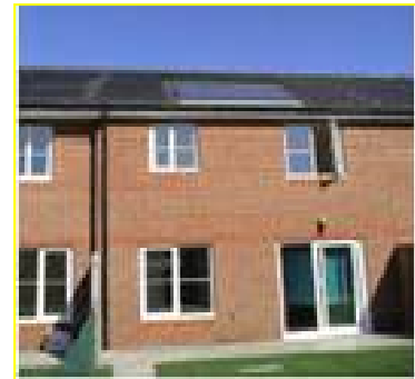
Contemporary design can capture passive solar gain and provide a strong image
