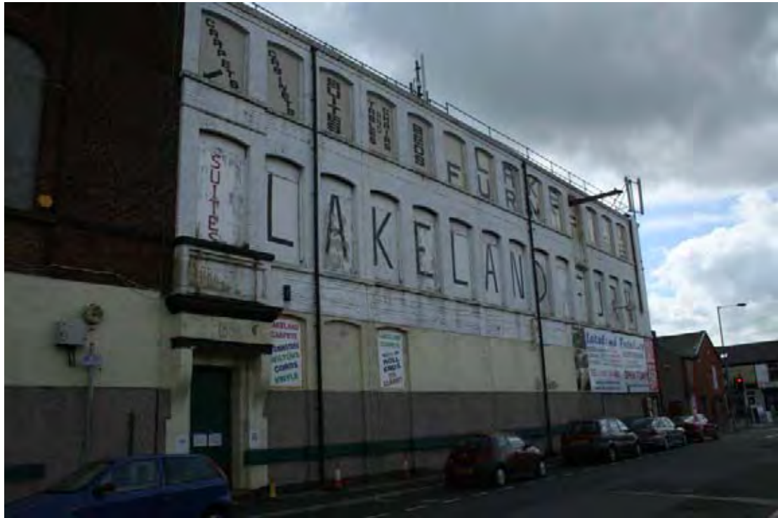
Plate 14 Former York Street Mill, Bury. Reused textile mill dated 1891, in an area recorded as Industrial works (general) (HER Ref HGM 10111)
