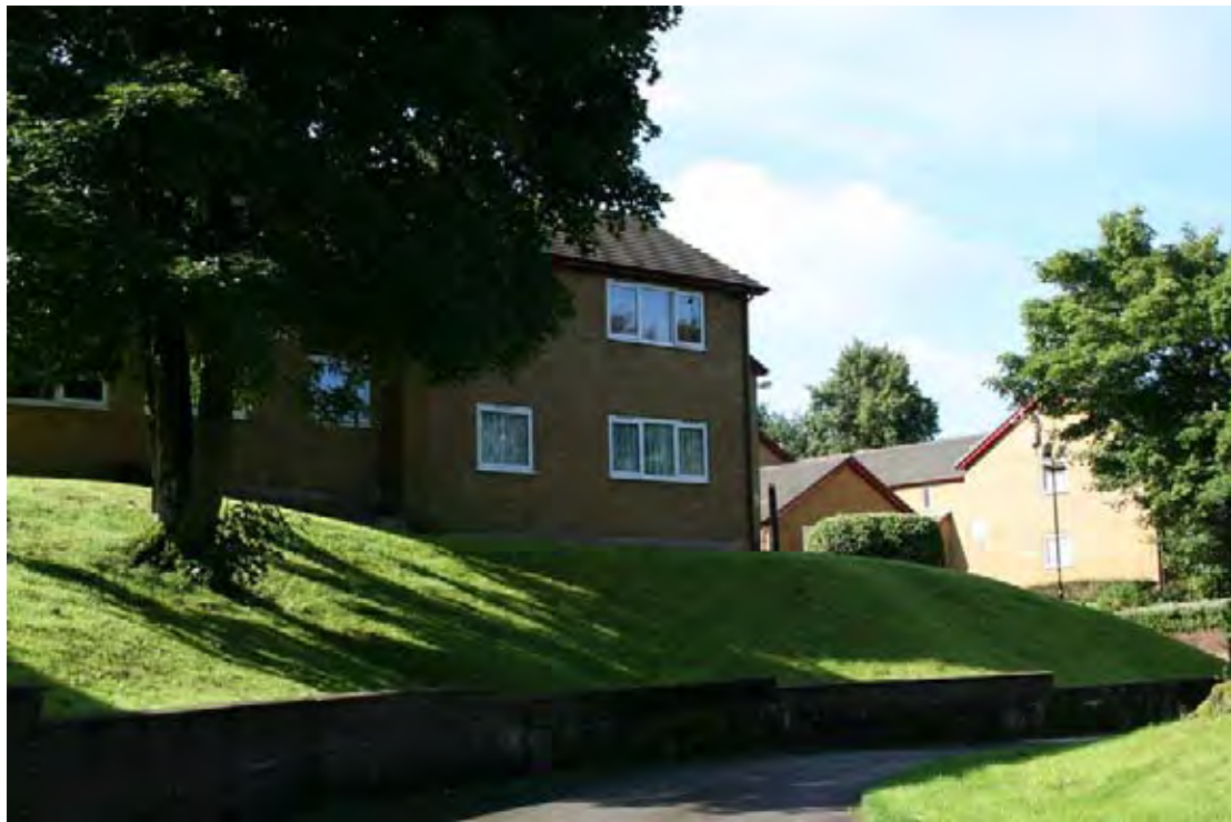
Plate 11 Low-rise flats – social housing of the later 20 th century. Off Clifton Road, Prestwich
