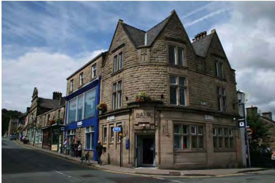
Plate 25 Bridge Street, Ramsbottom. Purpose-built late 19th century bank
