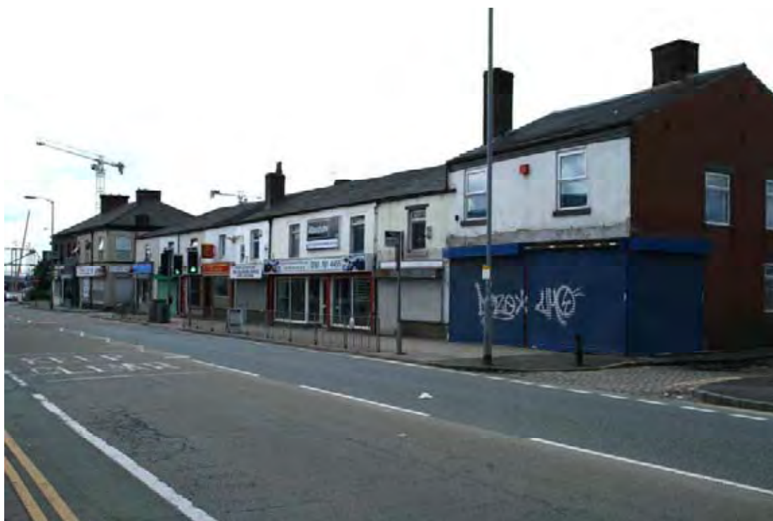
Plate 30 Walmersley Road, Bury. Pre-1851 commercial ribbon development
