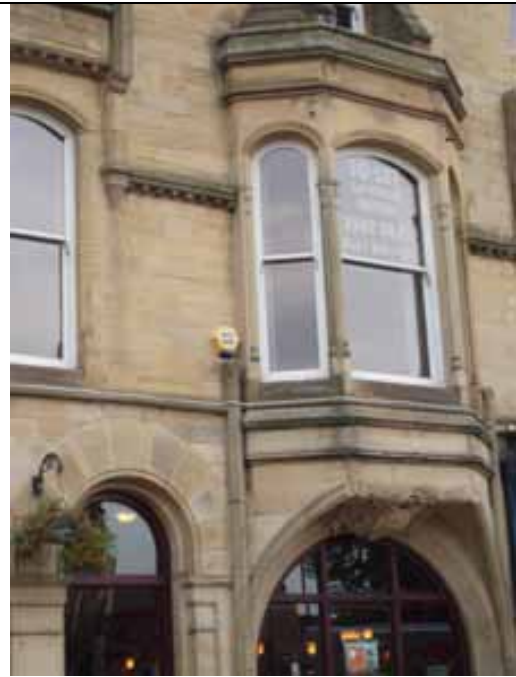
Fig. 111 Alarm box on Castle Buildings, Market Place
