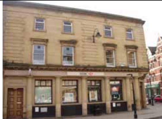
Fig. 100 Replacement upper floor windows, 2-4 Market Street
