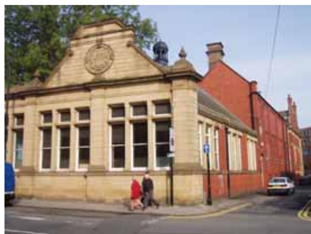
Fig. 35 Rear elevation of the School of Arts and Crafts School
