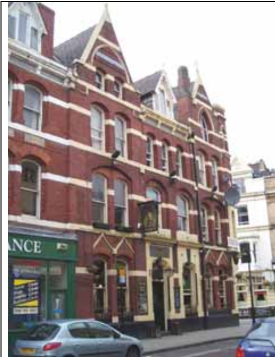
Fig. 110 Satellite dishes on the locally-listed Clarence PH on Bolton Street
