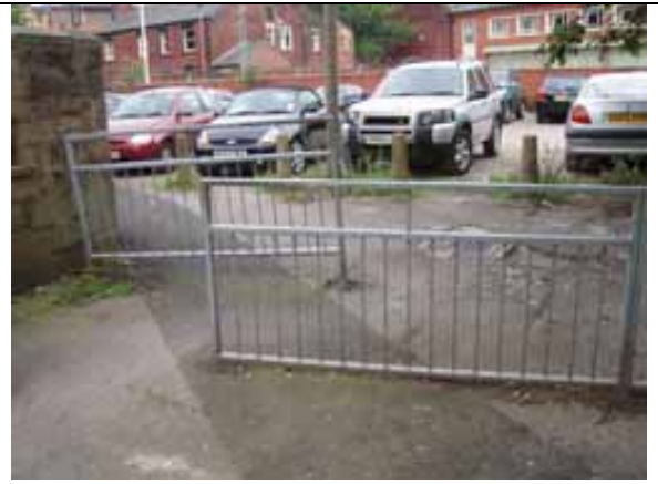
Fig. 130 Later twentieth century railings at the south end of School Brow
