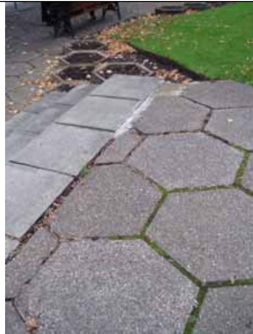
Fig. 78 Paving and planters, Memorial Gardens
