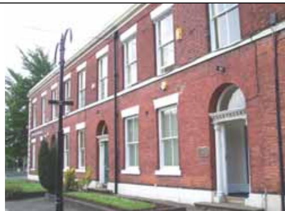
Fig. 60 Sash windows in (L-R) 14-10 Manchester Road
