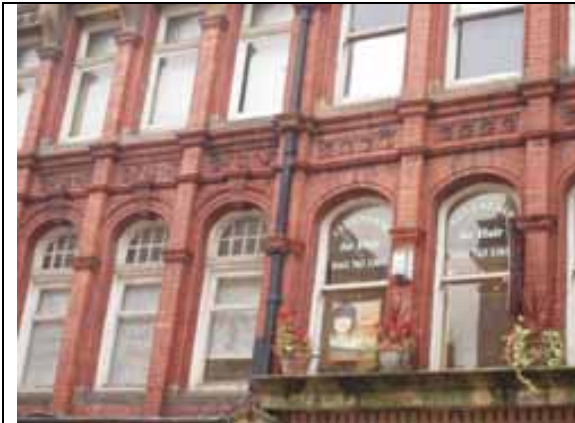
Fig. 58 Brickwork detail, 14-16 Silver Street
