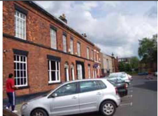
Fig. 103 Replacement windows in the listed terrace of St Mary's Place
