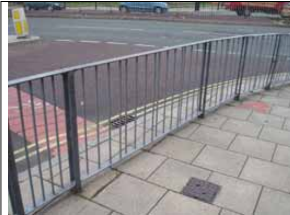
Fig. 129 Later twentieth century railings at the corner of Tenterden Road
