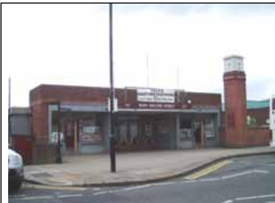
Fig. 23 Bolton Street station
