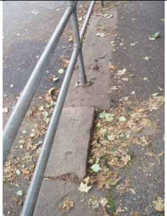
Fig. 81 Railings, School Brow (the old railing holes can still be seen)
