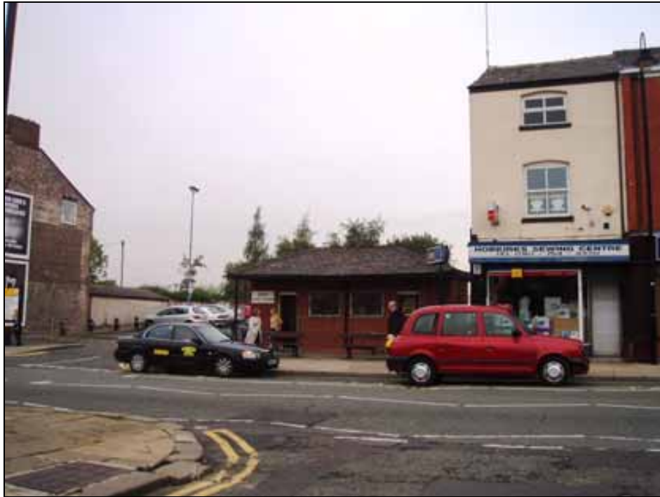
Fig. 114 Single-storey taxi office, Bolton Street.
