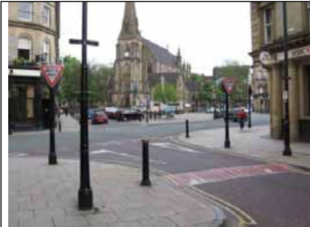
Fig. 126 Road treatment at the north end of Silver Street
