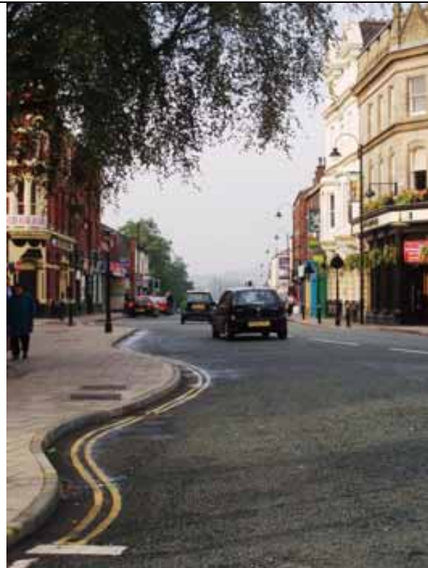
Fig. 86 Lamp standards on Bolton Street
