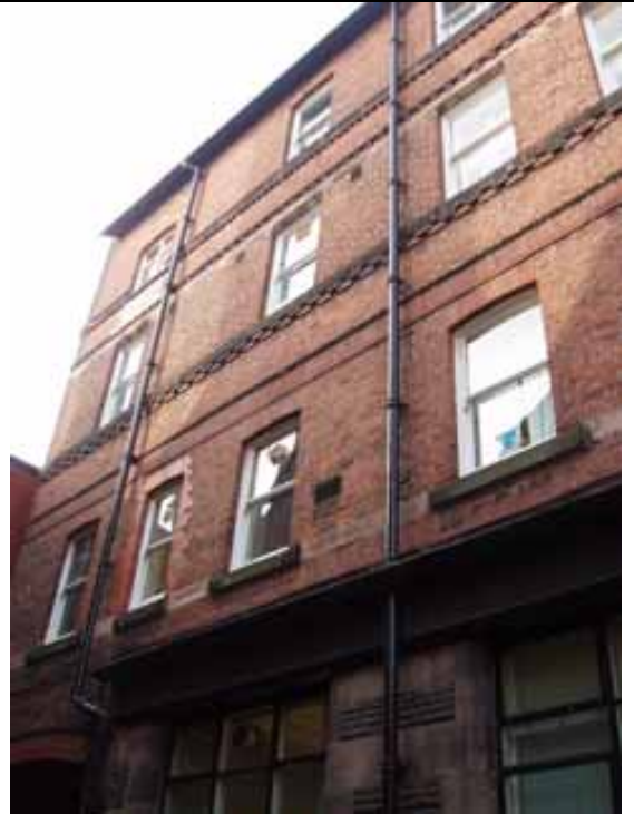
Fig. 65 Cast iron gutters to the rear of 21 Silver Street
