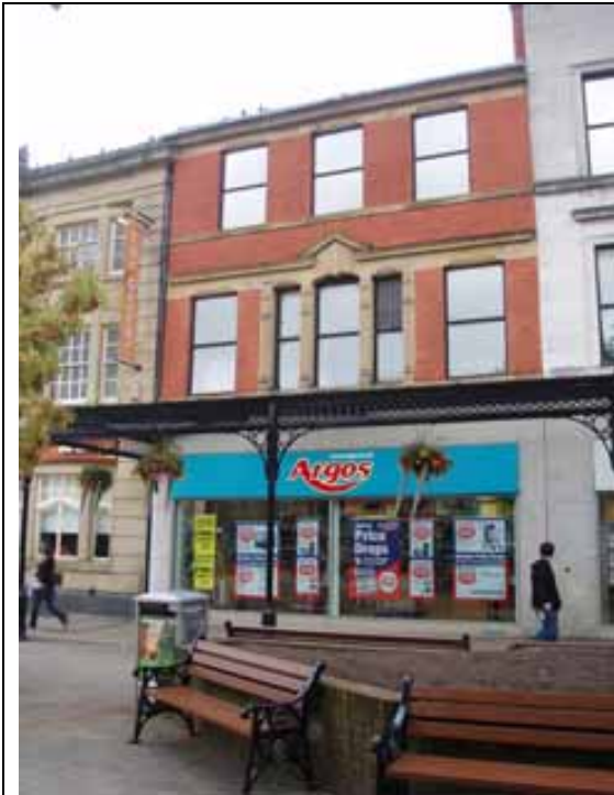
Fig. 104 Glazing replaced with mirrored glass, 6 Market Street
