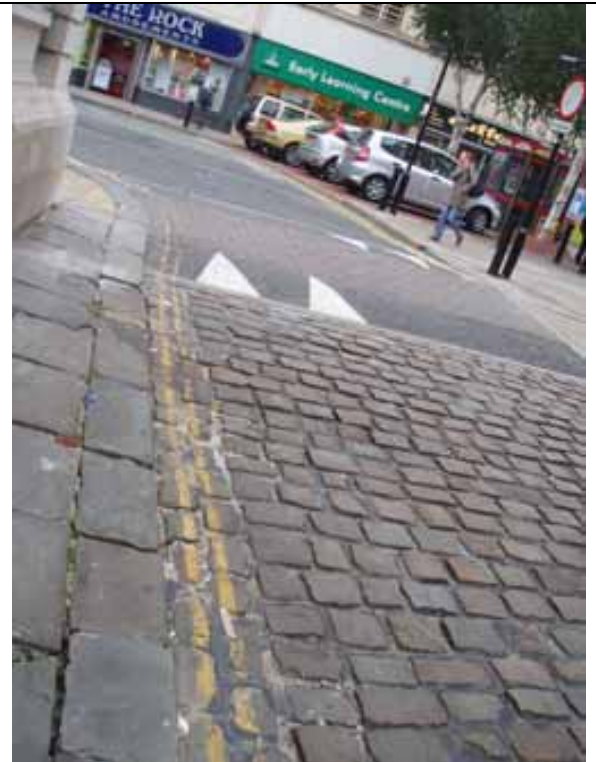
Fig. 72 Setts to north end of Gutter End
