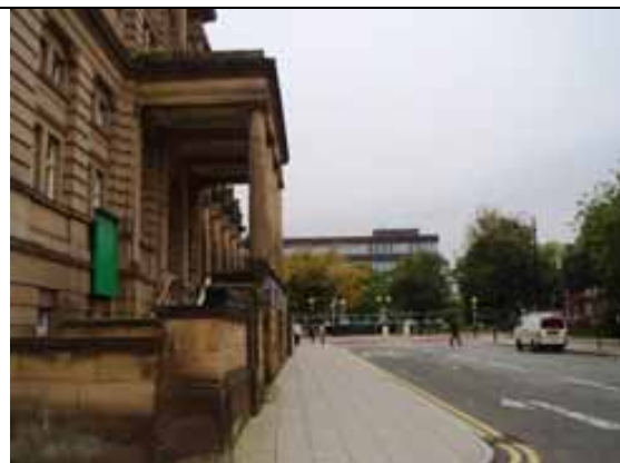
Fig. 93 View of Silver Street from Moss Street
