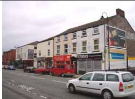
Fig. 101 PVC replacement windows, north side of Bolton Street
