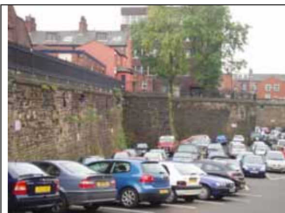
Fig. 25 Bolton Street station walls
