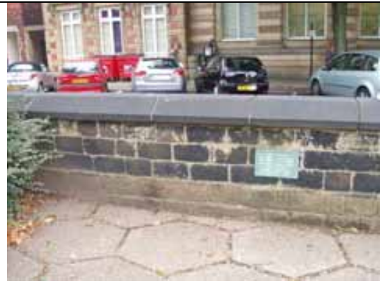
Fig. 59 Churchyard walls, Memorial Gardens, Silver Street
