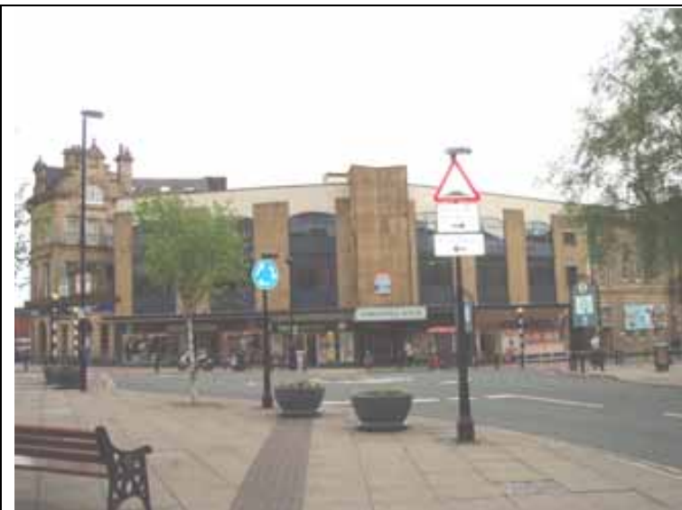
Fig. 128 Highways signage clutter on the corner of Market Place and Market Street
