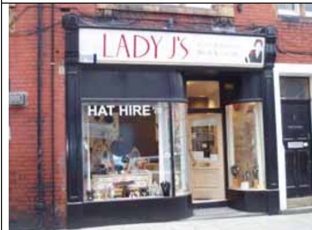
Fig. 69 Art deco style shop front, 1 Crompton Street
