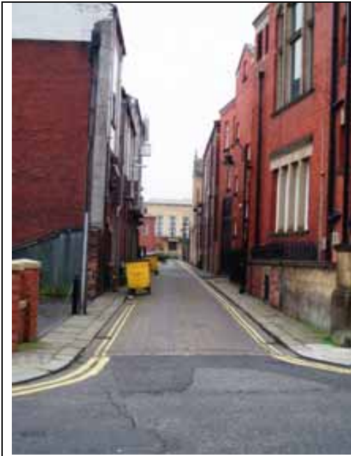
Fig. 42 View from Moss Street towards the town hall, beyond the conservation area boundary
