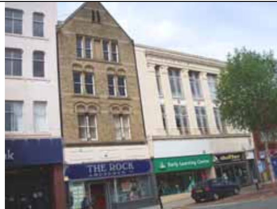
Fig. 109 Modern shop fronts, 13-21 The Rock
