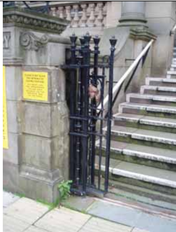
Fig. 63 Retracting gates, Bury Library
