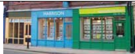
Fig. 21 Reproduction shop fronts on Bolton Street.
