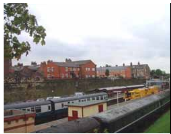
Fig. 8 Bolton Street station
