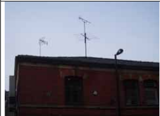
Fig. 112 Aerials on top of 18-20 Crompton Street
