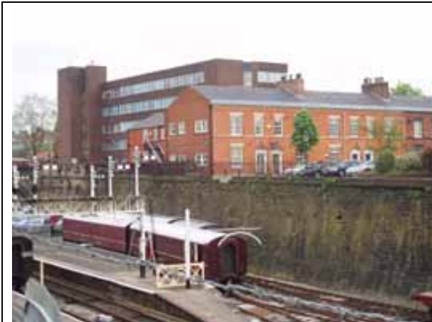
Fig. 9 Bolton Street station
