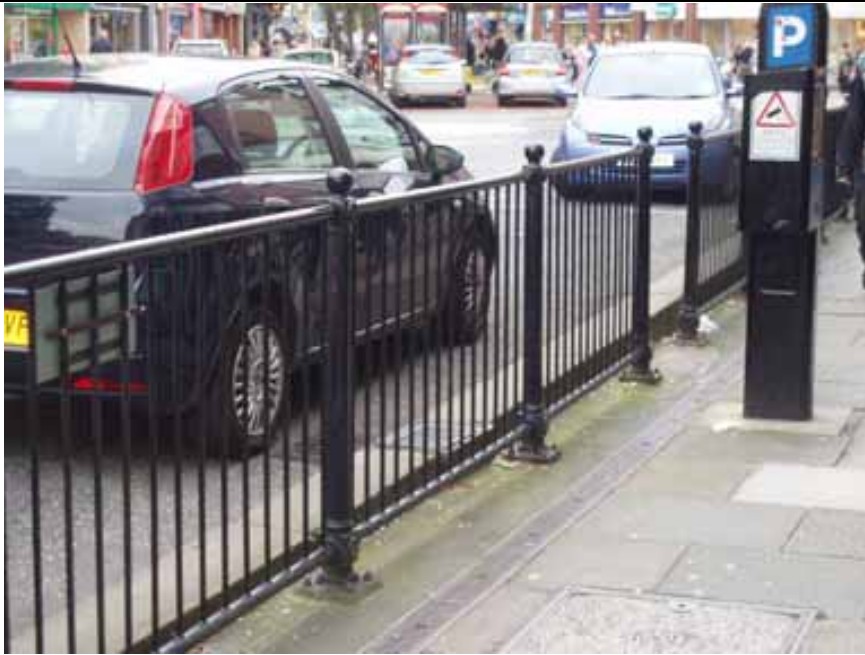
Fig. 84 Railings, The Rock.
