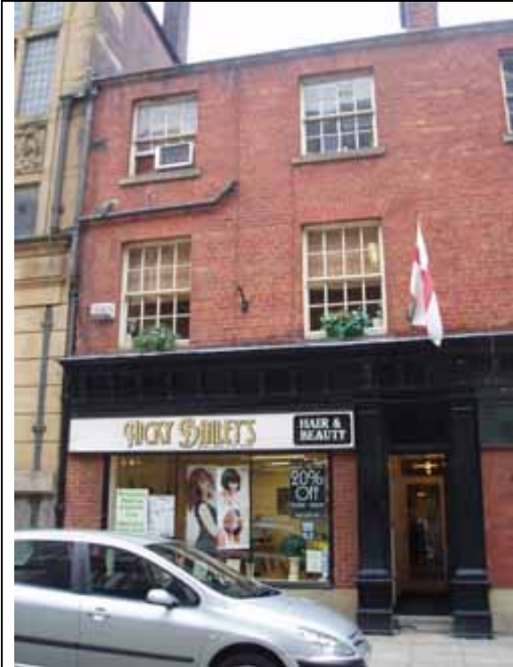
Fig. 64 Cast iron gutters on the frontage of 7 Broad Street
