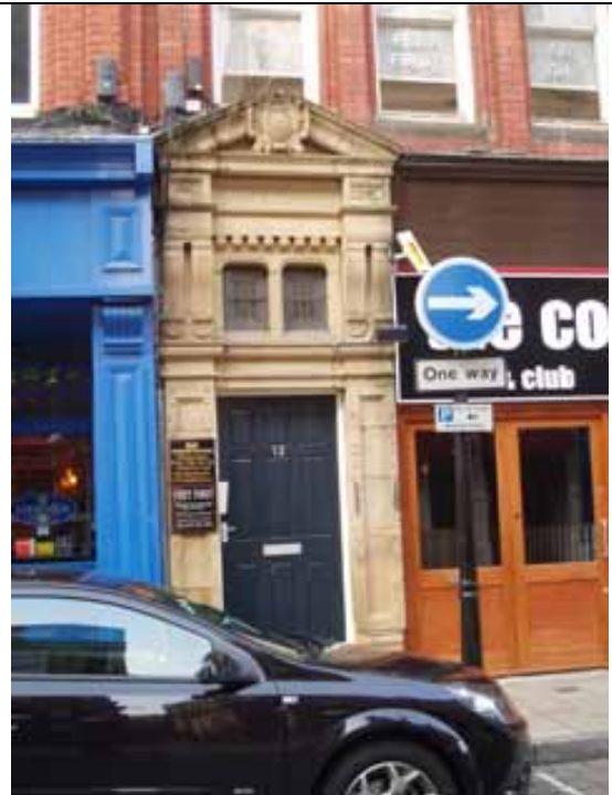
Fig. 55 Door case, Silver Street Chambers (1893)
