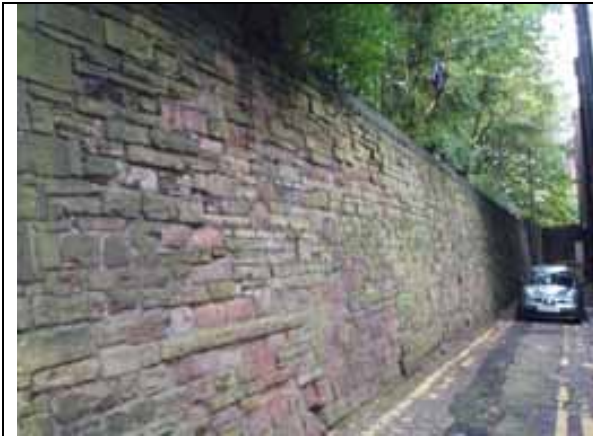
Fig. 16 Rectory wall, rear of 1 The Rock
