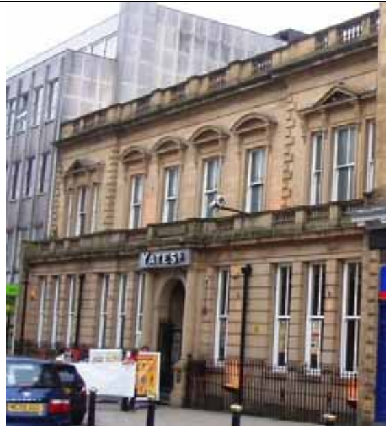
Fig. 102 Historic sashes, 20 Market Street
