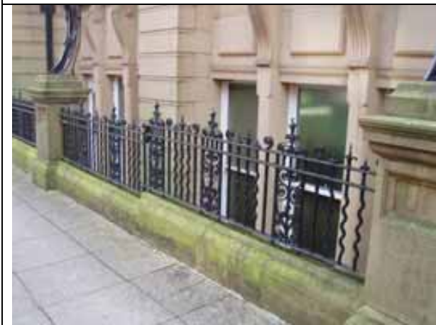
Fig. 82 Railings, School of Arts & Crafts
