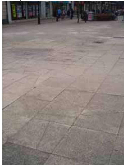
Fig. 77 Paving, Kay Gardens
