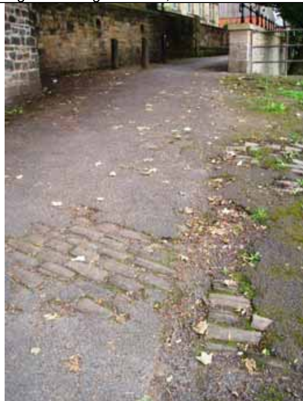
Fig. 73 Setts visible under tarmac, School Brow
