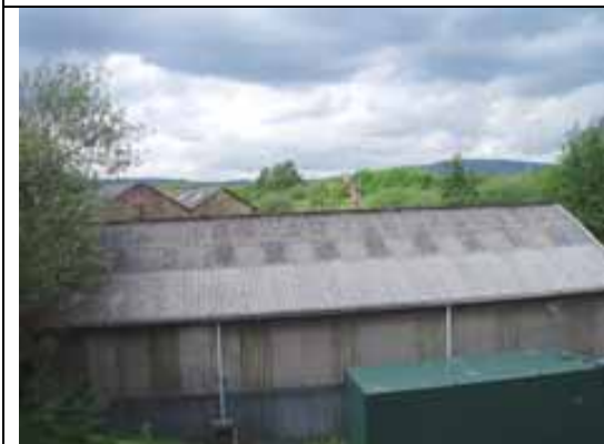
Fig. 123 Railway sheds opposite the west end of Castle Street
