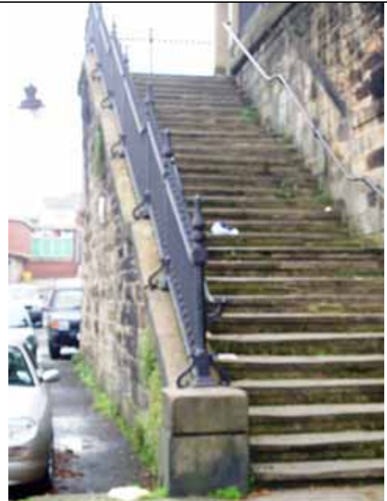
Fig. 10 Steps to Bolton Street station
