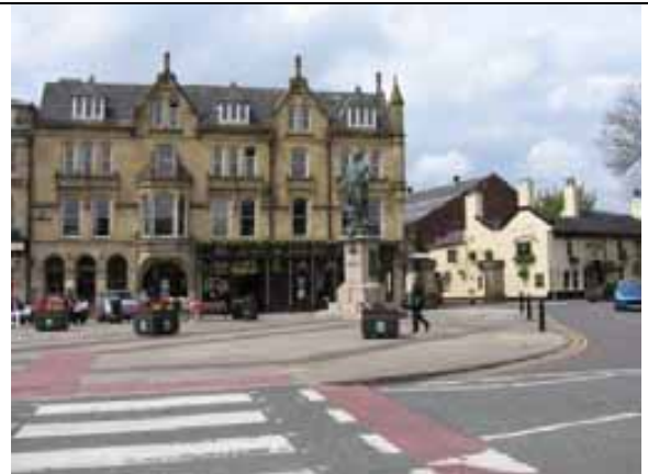
Fig. 127 Surfaces on the Market Place
