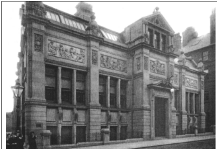
Fig. 44 Technical School, 1805 (Ashworth, 2002)
