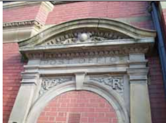
Fig. 56 Stone detail, former GPO, Crompton Street
