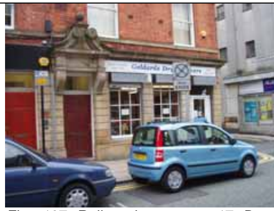
Fig. 107 Roller shutters on 17 Broad Street
