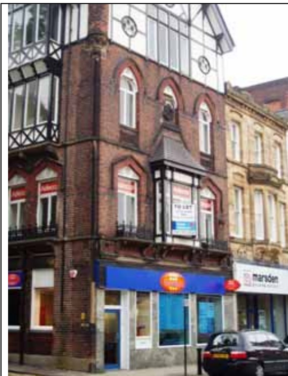
Fig. 117 To let: upper floors of 1 The Rock
