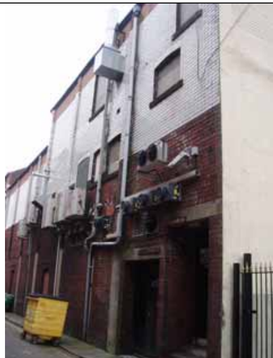
Fig. 135 Services to the rear of the Art Picture House, Haymarket Street
