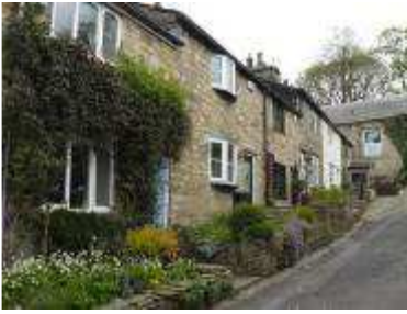
Windows on Hill Street
