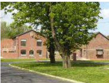
Tarmaced Driveway in New Development
