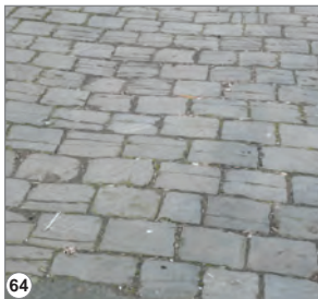
64) Setts on Church Lane.
