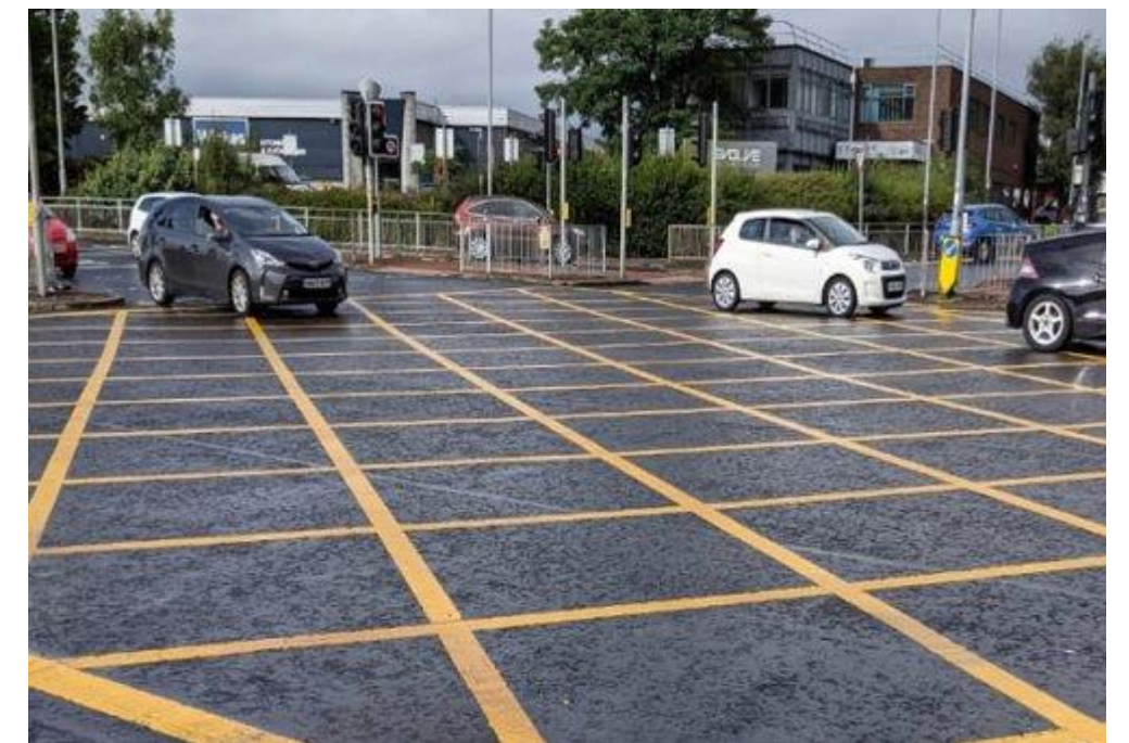
New Yellow Box Junction
