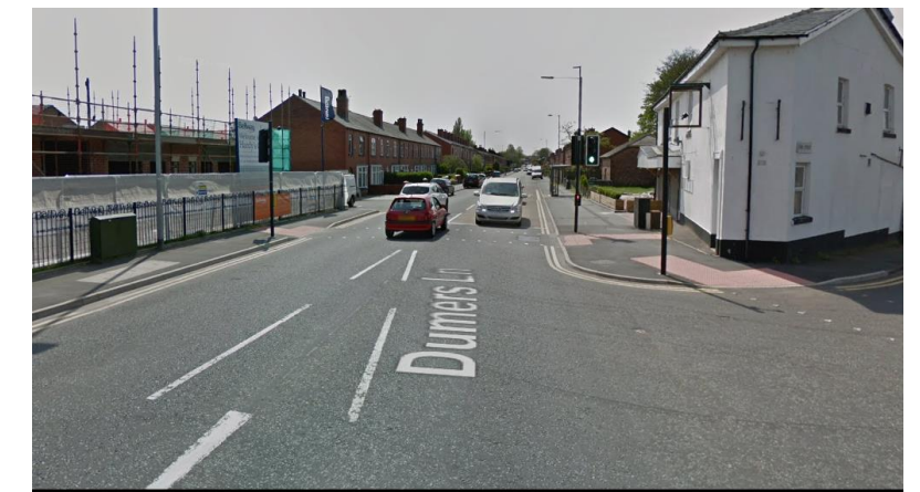
Dumers Lane before and after with pedestrian crossing facilities
