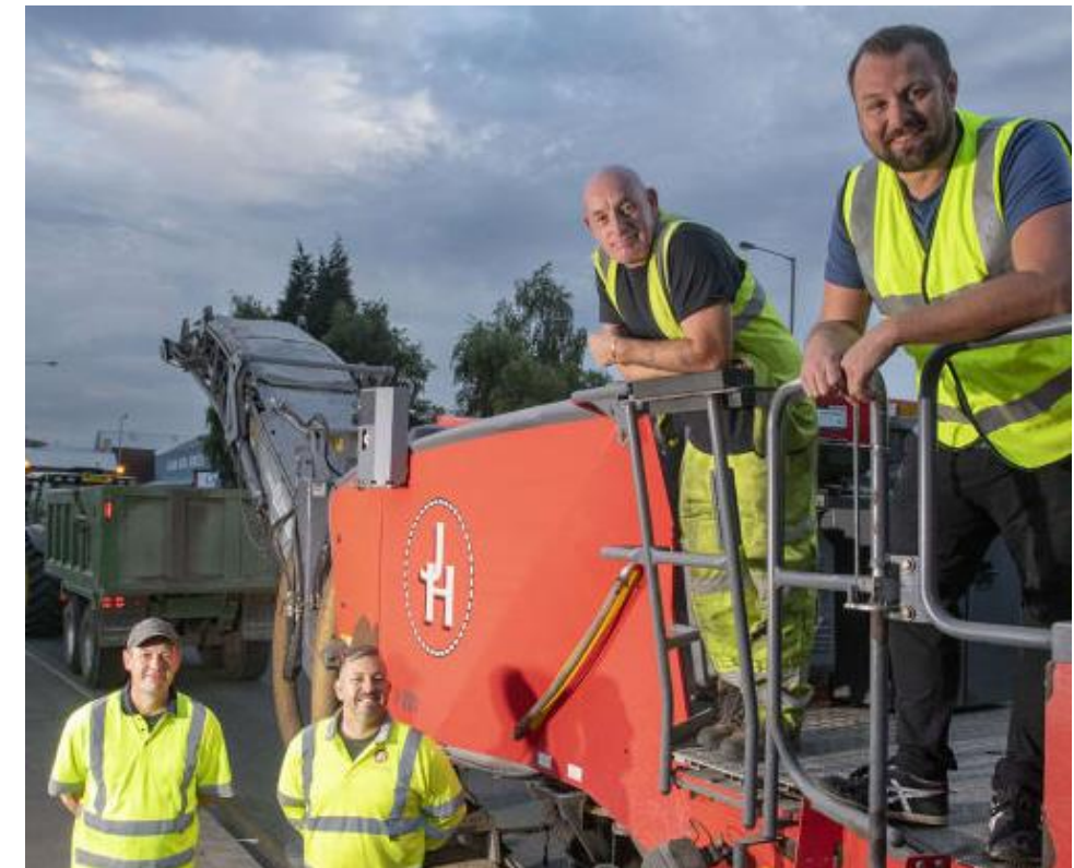
Resurfacing underway at Bury Bridge, Bury
