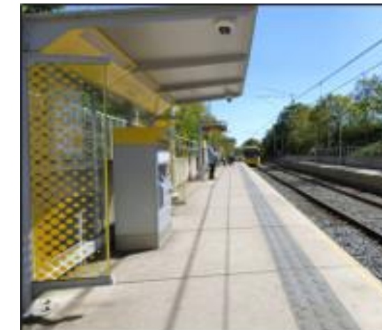
Firswood Stop - platform canopy
