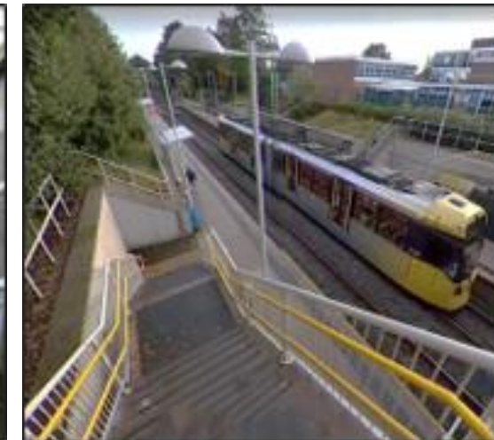
Firswood Stop - Step access
