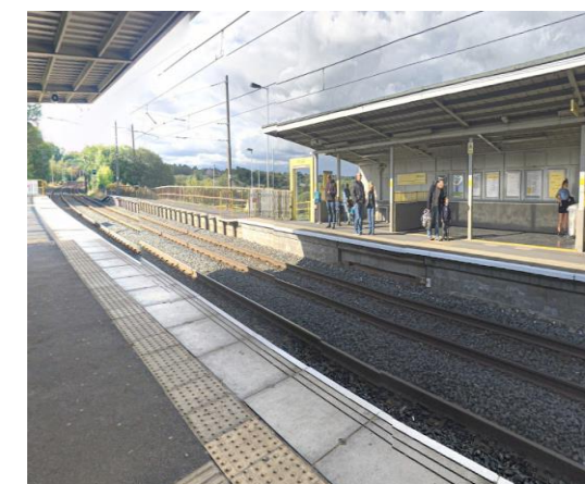
A typical Bury line track with no track crossing
