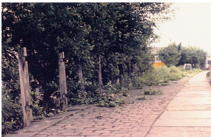
Ramsbottom Station before and after development
