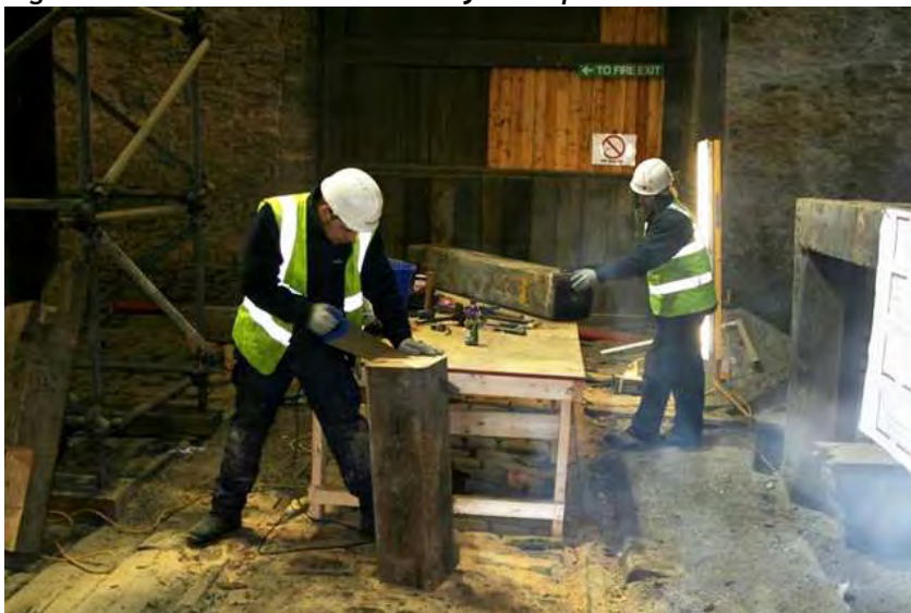
Figure 26: Restoration work at Bury Transport Museum
