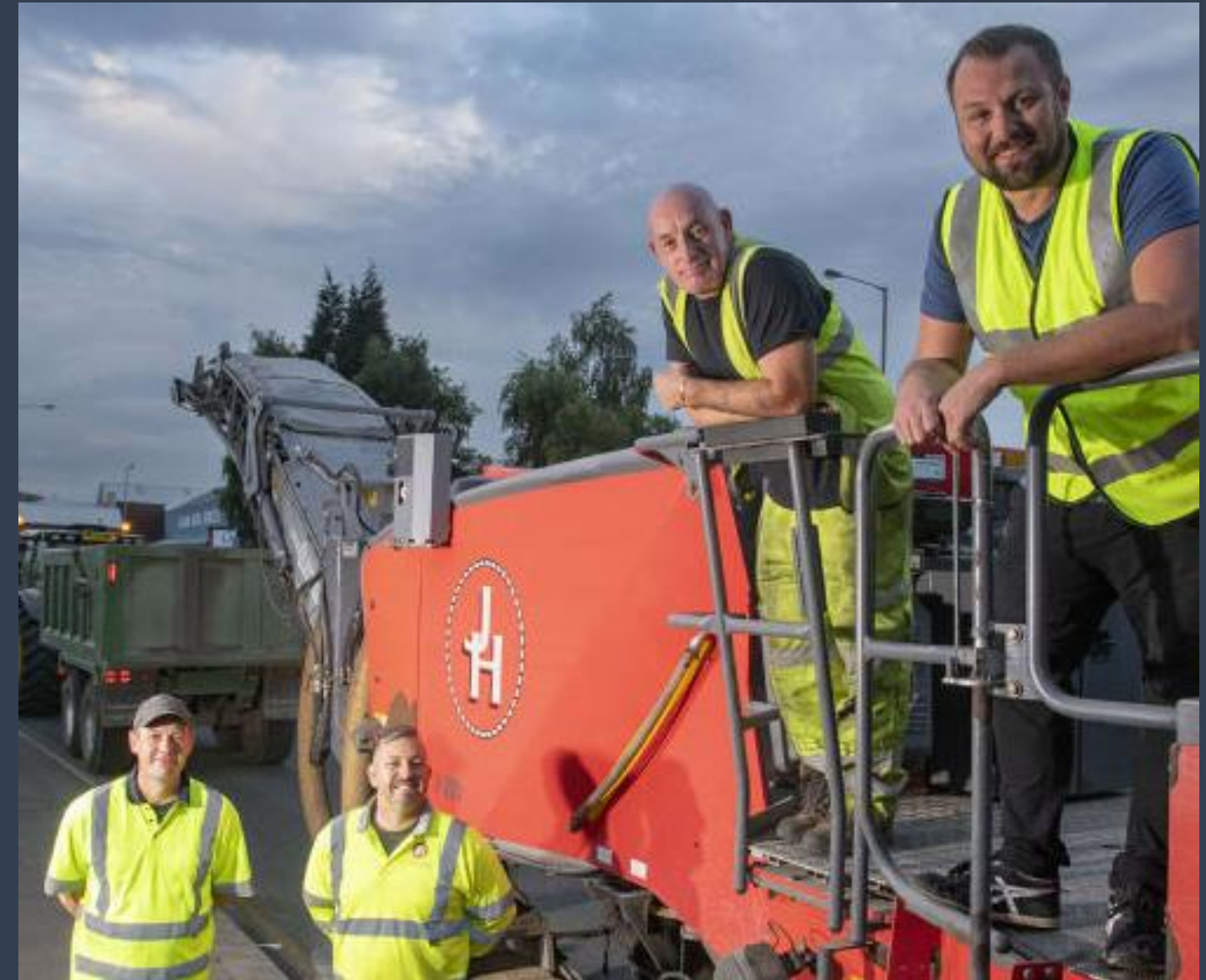
Resurfacing underway at Bury Bridge, Bury
