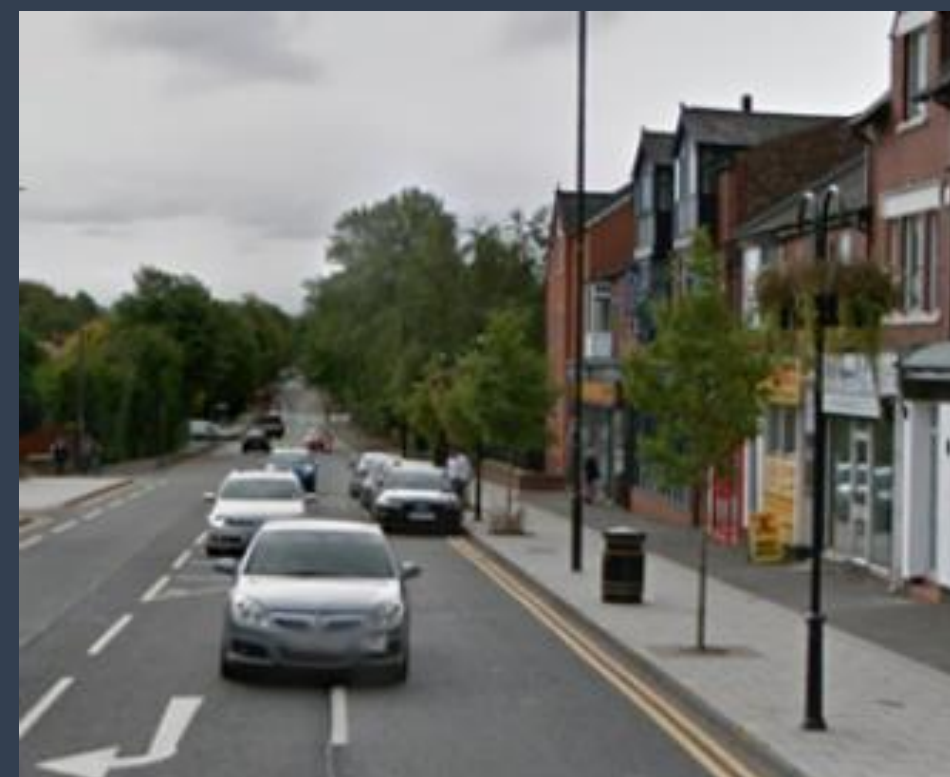
Prestwich High Street – After, SUDS drainage incorporated within tree pits
