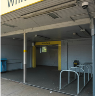
There is limited cycle parking provision at the tram station – and existing facilities are poorly overlooked
