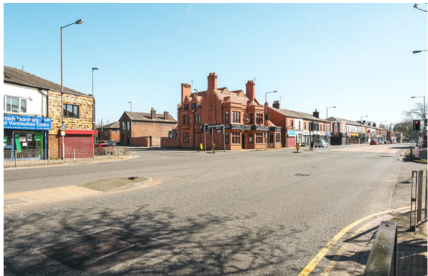
The junction at Bury New Road and Pinfold Lane / Moss Lane is also highlighted as an issue, with no signalised crossing, narrow footways and wide road carriageway.
