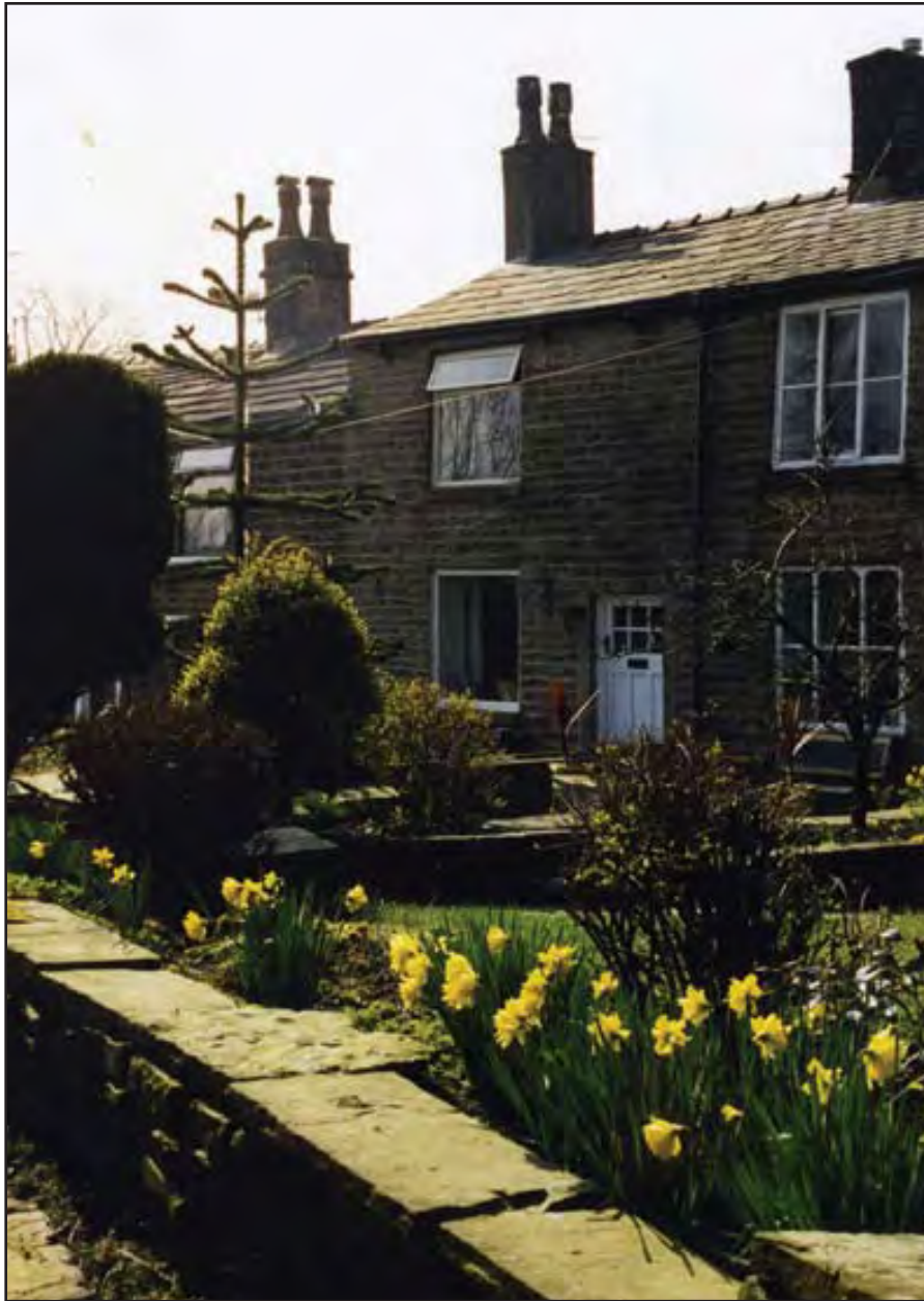
Club houses, top of Delph Lane
