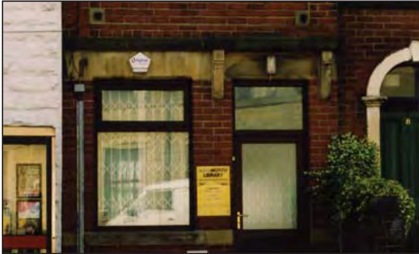
Library, showing later and darker red bricks, toning in with victorian terrace and contrasting with local stone of the pub
