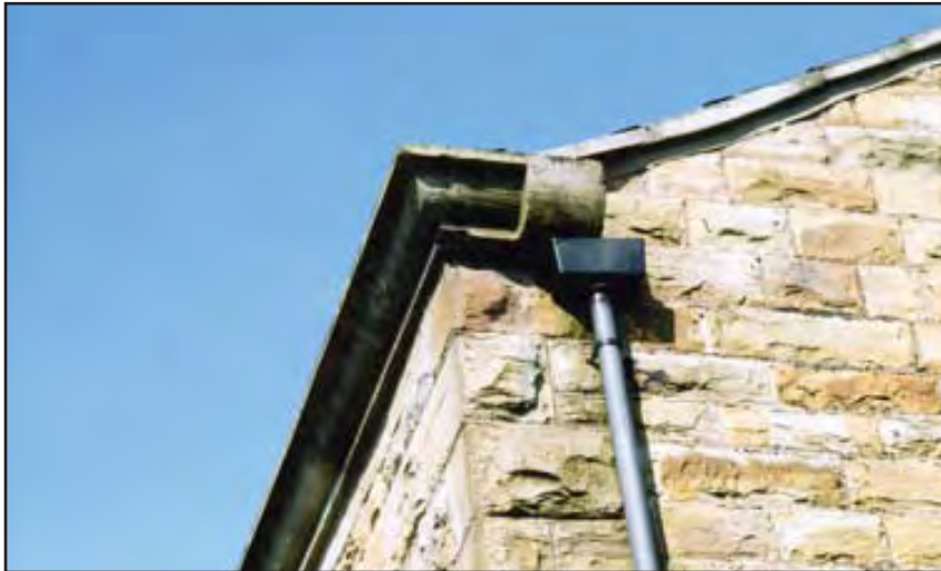
Plastic downspout on fine stone troughing
