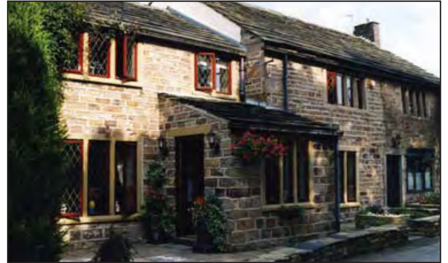
Local stone cottage, Ainsworth Hall Road, original ton slate roof, mullion windows sympathetically renovated
