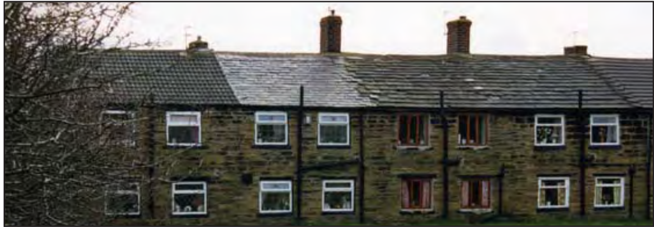
Local stone cottages, original ton slate roof, with reclaimed slate and modern concrete tiles at Hulmes Terrace
