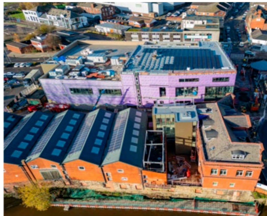
Radcliffe Hub (in construction)
