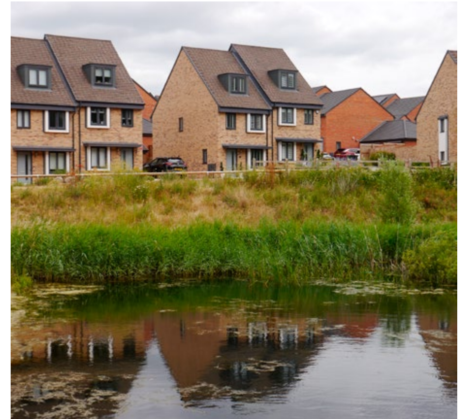
Example of drainage feature
