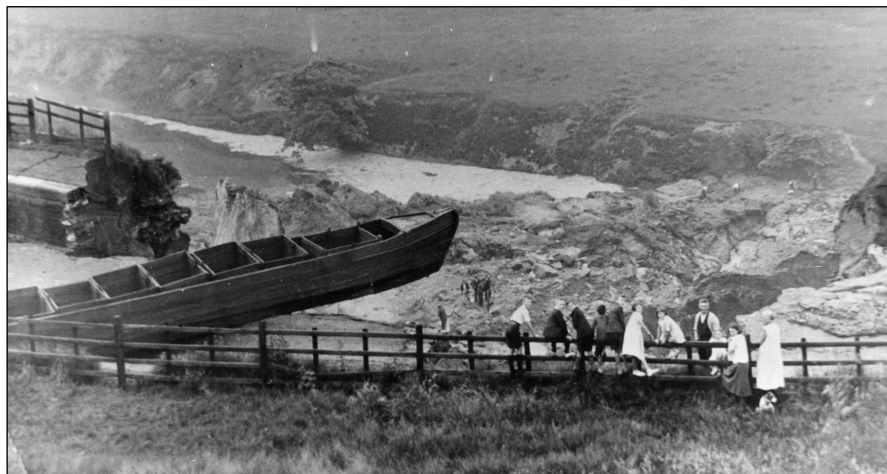
Figure 9 – The 1936 Manchester, Bolton and Bury Canal Breach
