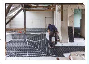
surfaces! This gives you a good range of design options and also is a good solution for the cold, unforgiving nature of stone floor. However, be careful of the set up costs. Generally it's better to install your underfloor heating system to coincide with getting a new floor or other updates.
